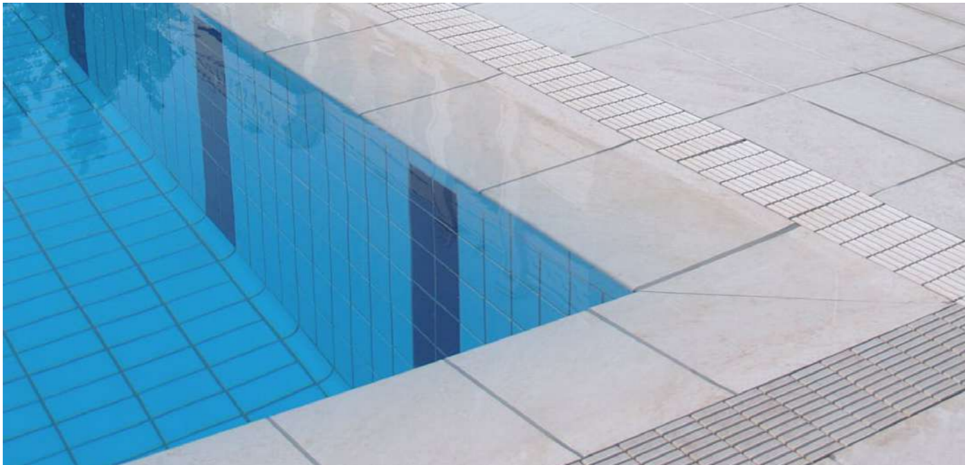
Rehabilitación de piscina comunitaria con borde 500 Beige Stone. Restoration of community pool with 500 Beige Stone border.
